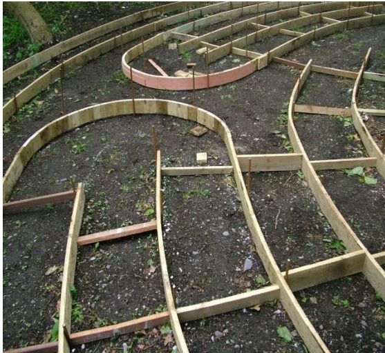
Above: Walls of the labyrinth being constructed and pinned down
